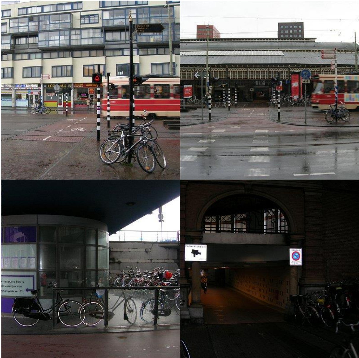
One of the many projects in The Hague: new tunnel for cyclists and pedestrians under main railway station. Complicated project regarding social safety (tunnel structure) and traffic safety (tram crossings).
